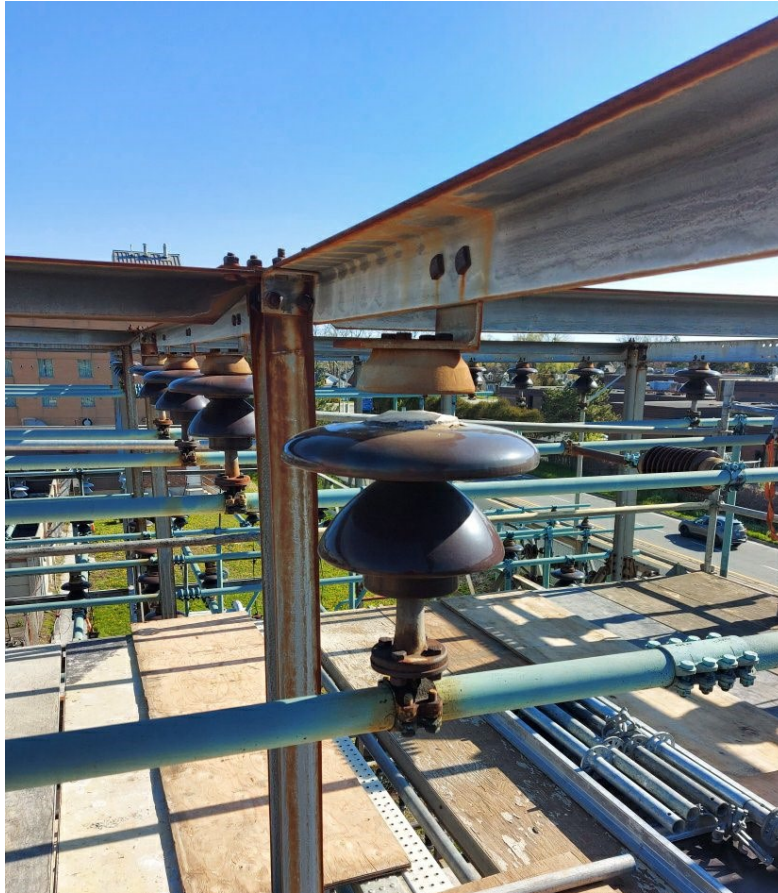
Crews replaced aging infrastructure, including insulators seen above.
