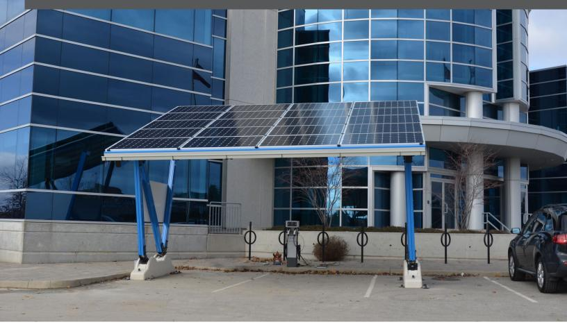
A lectra Utilities was one of the first utilities of its size in North America to build a proof-of-concept microgrid. Alectra's microgrid, at its office in Vaughan, Ontario, works like the electricity distribution grid, but instead of delivering electricity to hundreds of thousands of customers at a time, it is scalable to service targeted customers — in this case, Alectra's Vaughan office.
